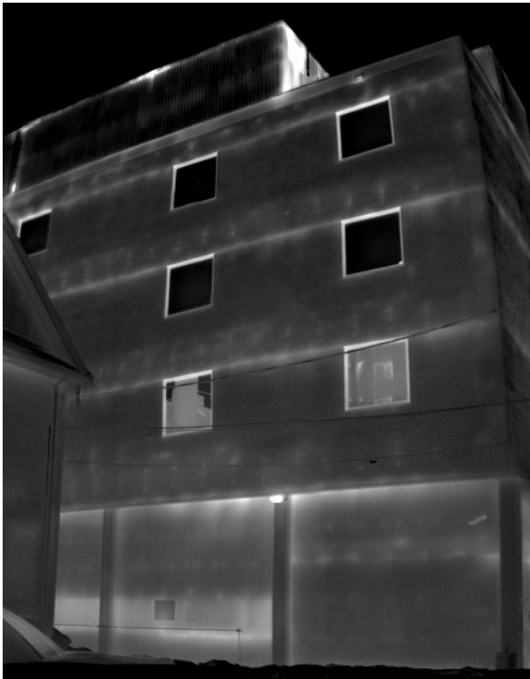
Figure 19. Negative Building Pressure (-8 Pa), To =-11 °C (12.2 °F)
